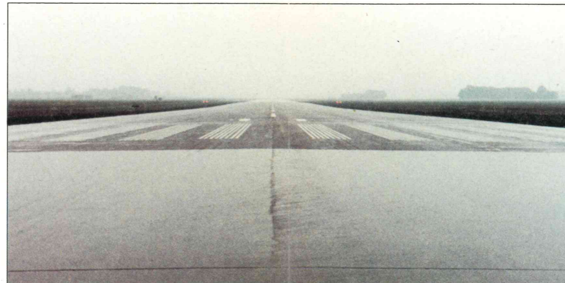
The grooved part of the runway is almost dry when the non-grooved part is covered by a sheet of water.
